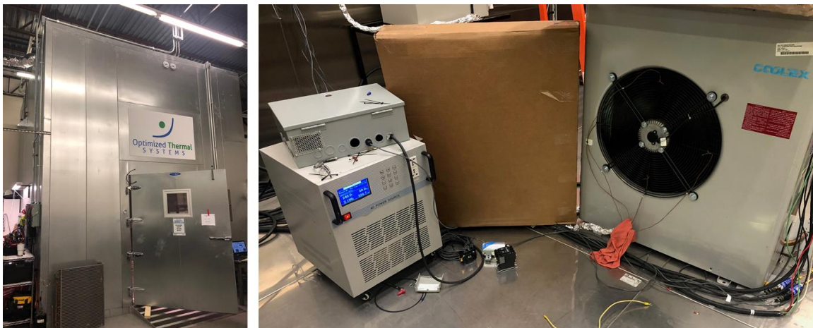
Figure 20. OTS Setup: outdoor chamber (left), Unit 10 and frequency converter inside chamber (right).
